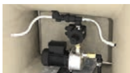
Pump installed with rain/mains changeover (sits behind door)
